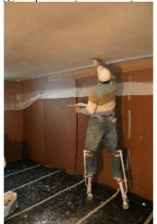
Next they added the sister joists. Finally, they put the ceiling back up. Master plasterer Steve and his assistant Henry replastered the ceiling in two hours. With a fresh coat of paint applied only two weeks after we began, we are ready to show off this restored ceiling when we reopen for tours on Patriots Day.
