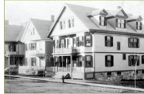
Wooden sidewalk on Bowker Street, date unknown.
