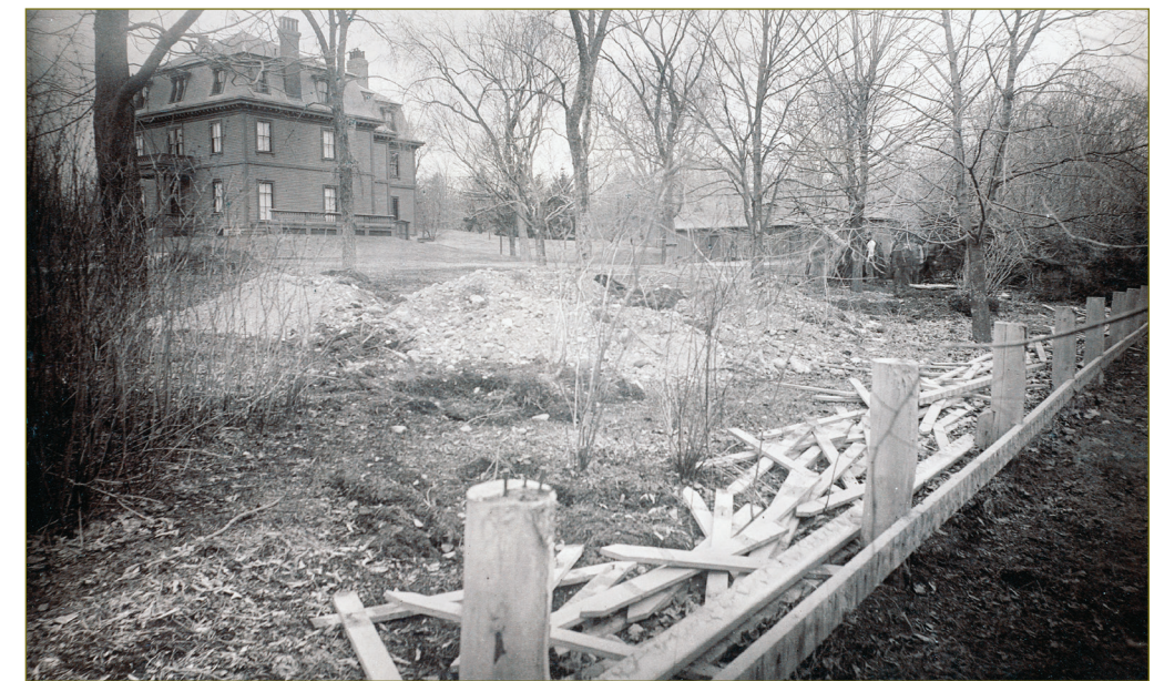
Workers removing the fence and trees of the Charles Cotting house, still standing on Hawes Street. (Digital Commonwealth [CC BY-NC-ND]. Brookline Photograph Collection published by the Public Library of Brookline)
